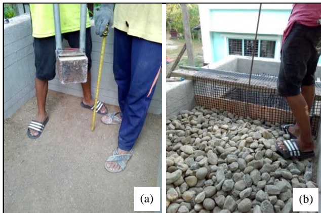
Figure 9. Soil compaction (a) and gravel rodding (b)
