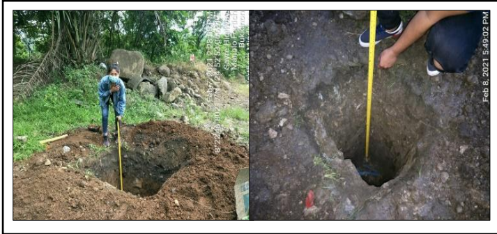
Figure 1. Measuring the depth of the excavation
