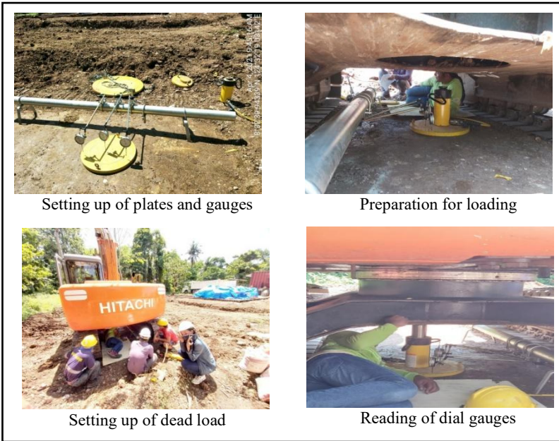
Figure 6. Plate load testing of samples
