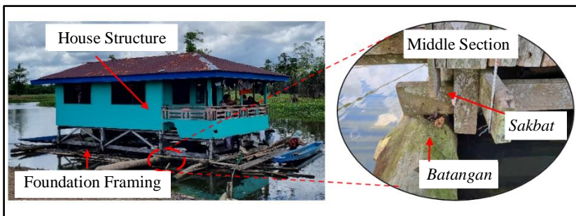
Figure 6. Structural components of the foundation framing and the house section
