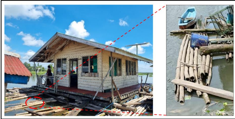
Figure 5. Floater using bundled bamboo ( Batang )
