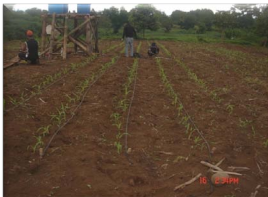
Figure 1. Drip installation in the area
