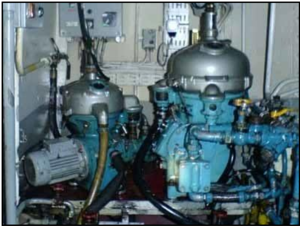
Figure 2. Marine fuel preheating and purification system
